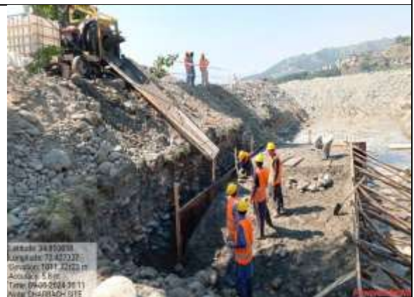
Local labor with PPEs at Charbagh Site Swat
