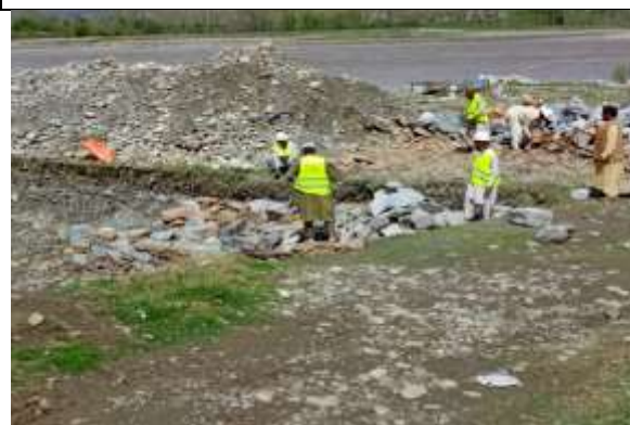
Labor Working at Package 13 and 14 along Swat River with PPEs
