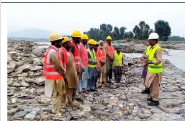
Safety Meeting with Labor at site at package 13 & 14
