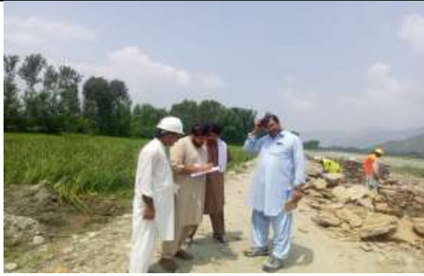
Filling Environmental Compliance Checklist during Site Visit at Jalawanan Site
