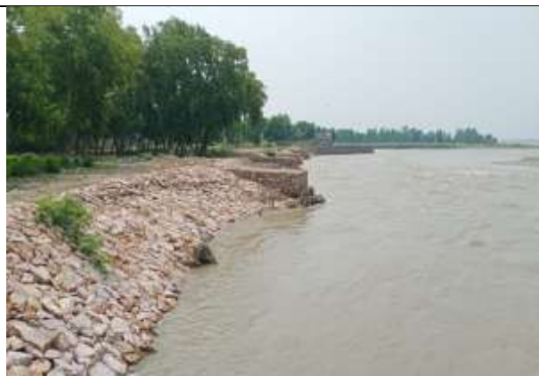
Gabion Wall Works at Dhaggi Faizaulah (Package 11)
