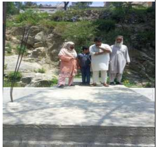
Visit to Footbridges at Shalfalam
